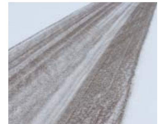
The above photograph shows the pattern formed directly after the dispersal of moist grit
